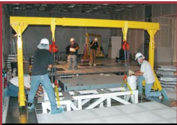
Cleanroom Rigging & Installations
