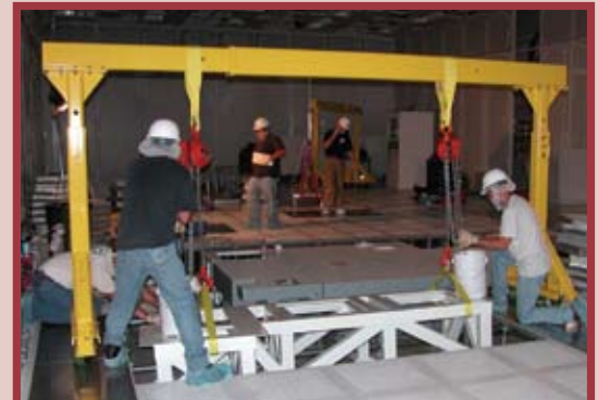
Cleanroom Rigging & Installations
