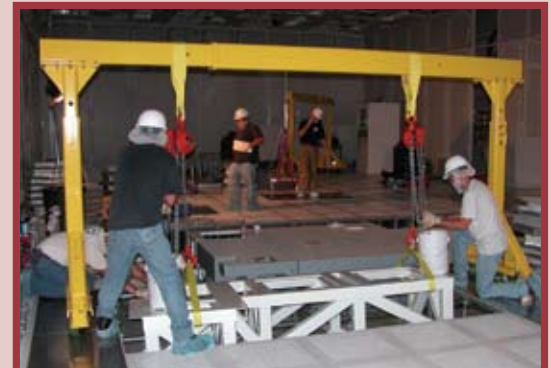
Cleanroom Rigging & Installations
